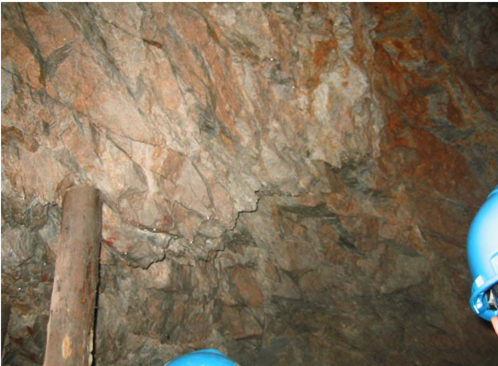
Figure 6: Timber Used as Ground Support in Tarzan Gold Mine
