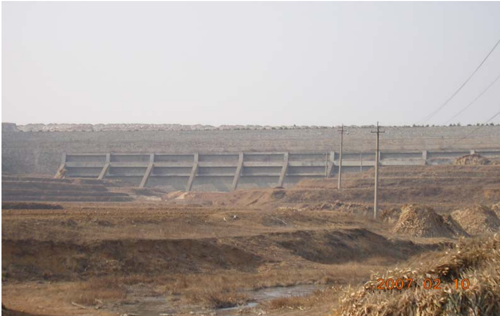
Figure 1: Tailings Dam for Yingezhuag Gold Mine
